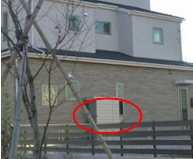
A. Installation at private house
